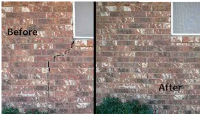
Before and After Foundation Repair
