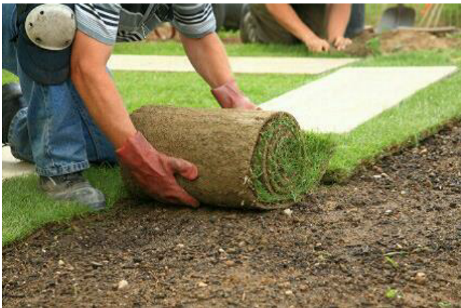
Install New Sod 100% Kentucky Glue Grass
