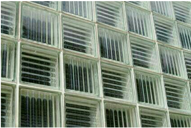
Example of glass block windows
