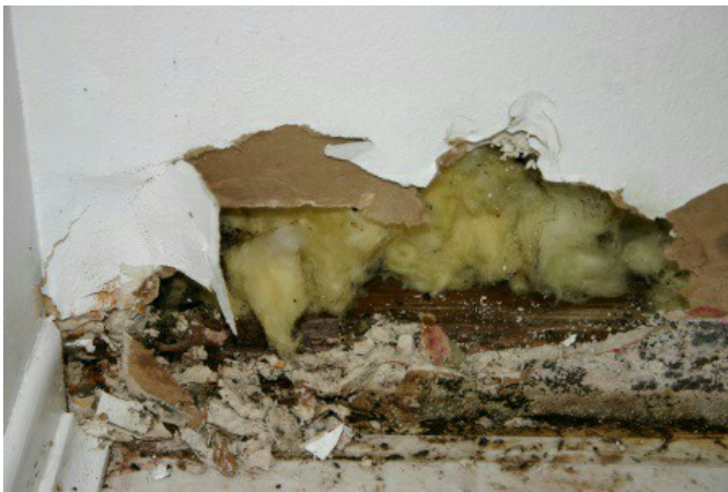
Mold and water damage in basement on bathroom wall
