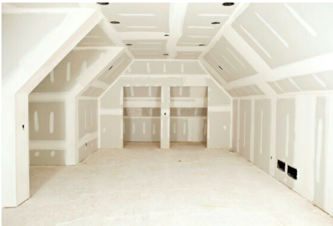
Example of completed drywall work from previous home
