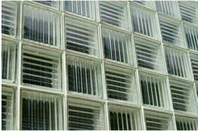
Example of glass block windows
