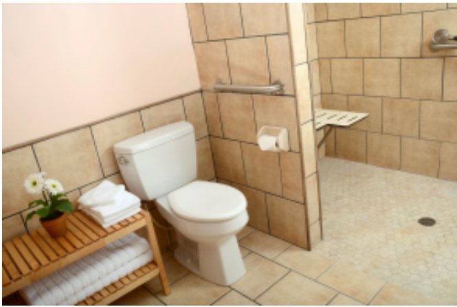
Example of previous barrier free shower installed
